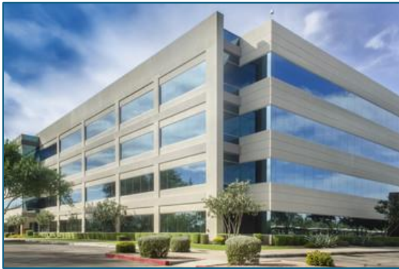
Figure 39: Standalone office building. Source: BCFC via Adobe Stock (n.d.).
