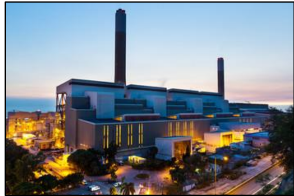
Figure 44: Cement plant. Source: leungchopan via Adobe Stock (n.d.).
