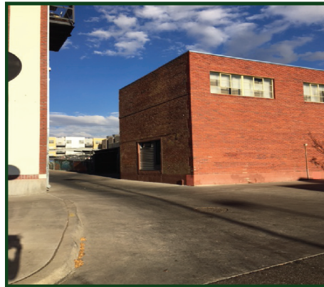
Alley Entrance from 25th
