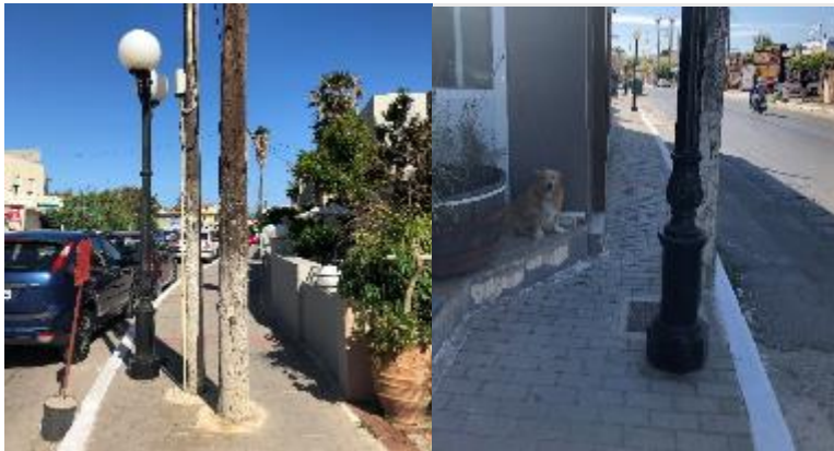
Figure 26. Sidewalk obstructions: Utility poles and street lamps
