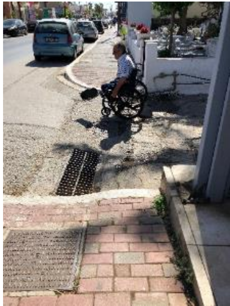
Figure 27. Stormwater grates, steep slopes and high curbs present obstacles for people with mobility challenges
