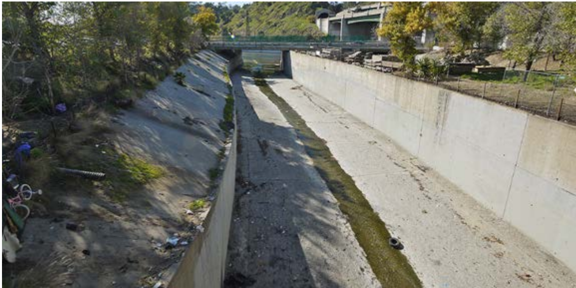
Figure 84. Water channel in Los Angeles, California similar to Stalos channels
