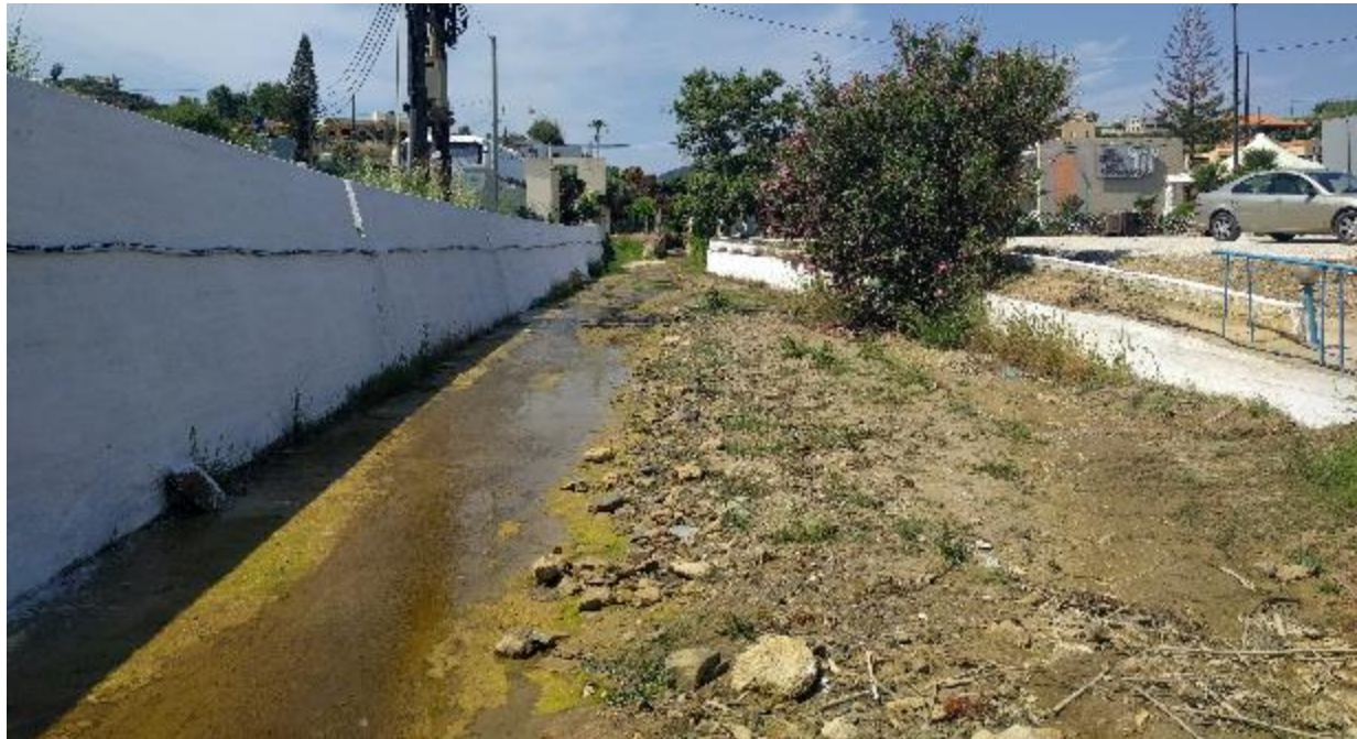
Figure 83. Existing upstream concrete channel
