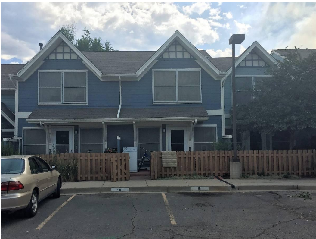
Figure 55. Appliance and household items on the porch of a Woodlands residence; pavement damage
