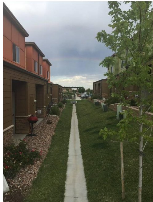
Figure 15. Storm water drainage between the rows of townhomes
