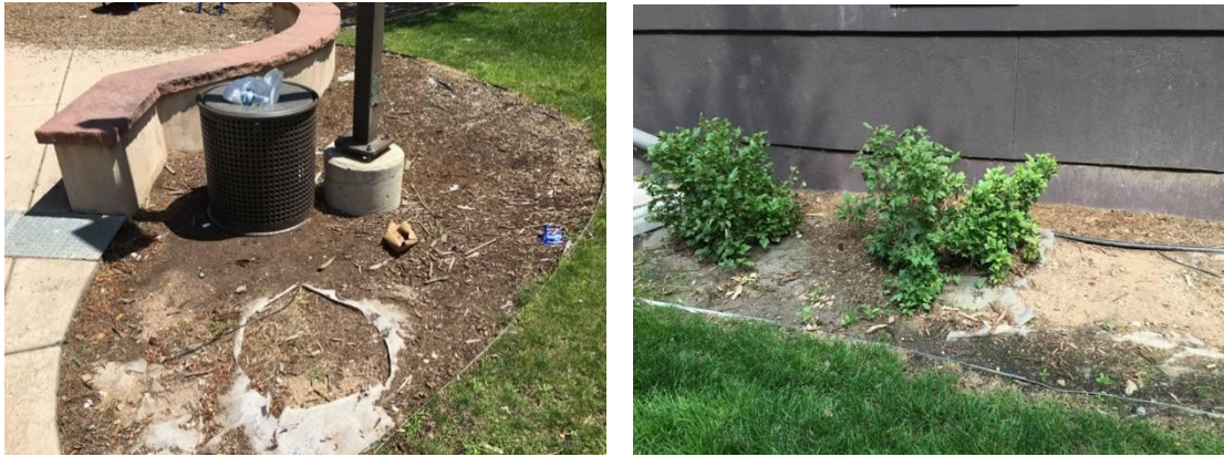
Figure 24. Overflowing trash receptacle, minor litter, and worn landscaping
